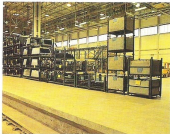
Pallet unloading area
